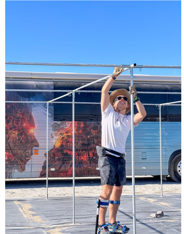
Drywall stilts are cheap, easy to use, and make it much faster to install tarps
